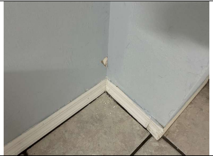
HM-A: Drywall/Joint Compound, White
